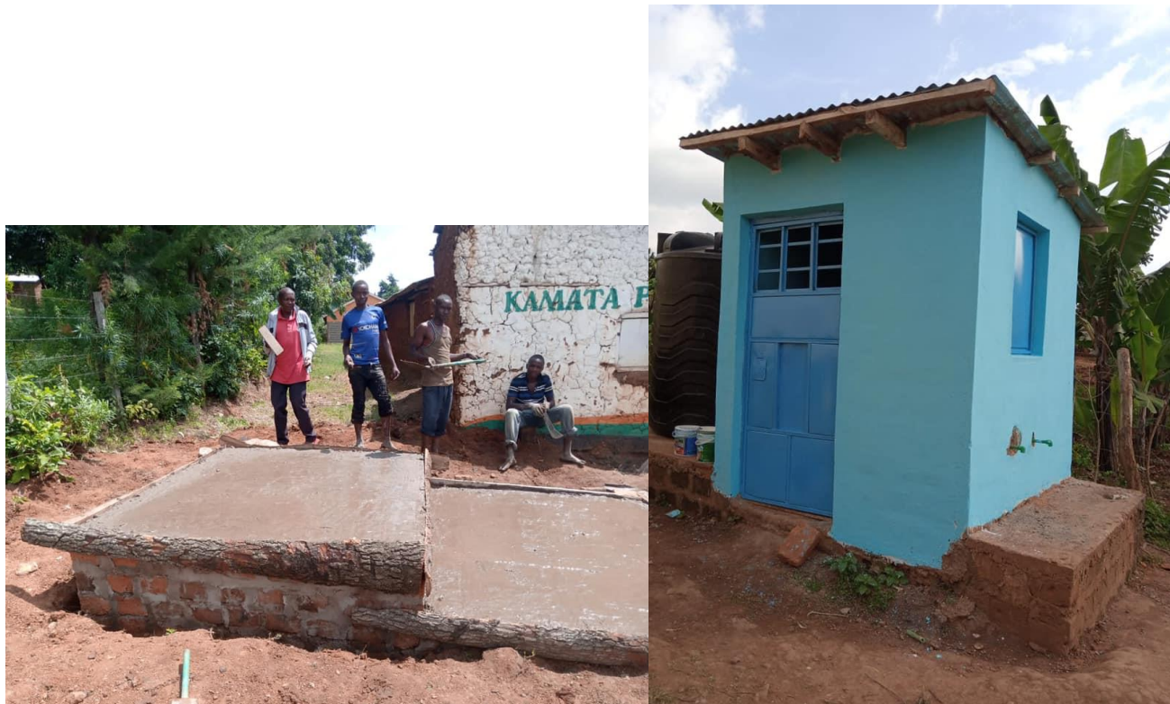
Foundation base for the water kiosk at Kamataa Primary School (left). An almost complete water kiosk at Peresten Primary School (right).
