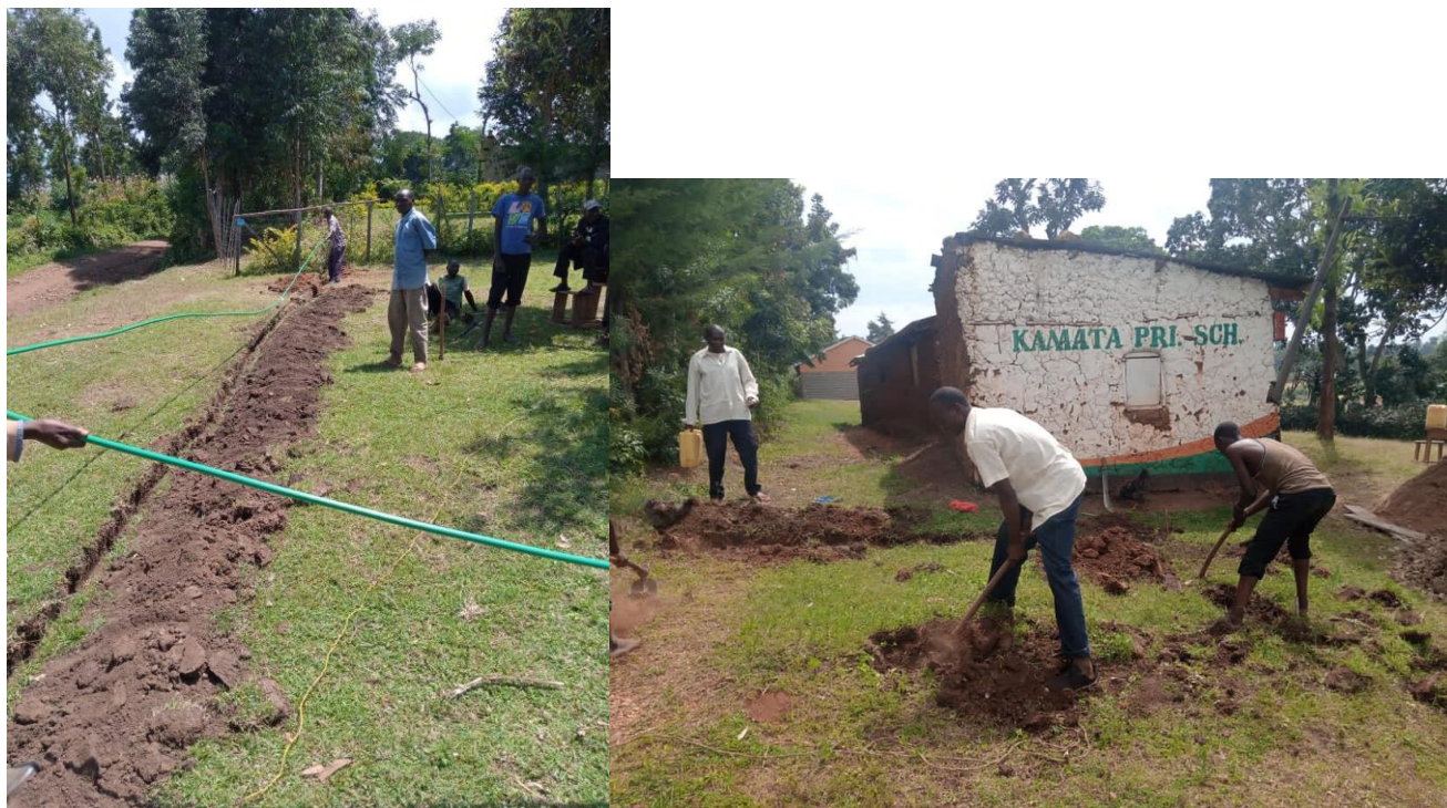
Community residents laying down of pipes and digging for foundation base for the Water Kiosk at Kamataa Primary School.
